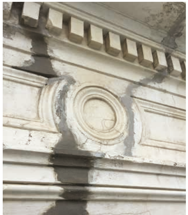
Detail of facade restoration works, South Melbourne Temperance Hall ►
